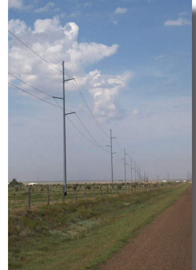
Transmission Line Rebuild
