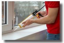
frames, baseboards, and around pipe inlets too (particularly pay close attention to pipes underneath sinks on exterior walls).
